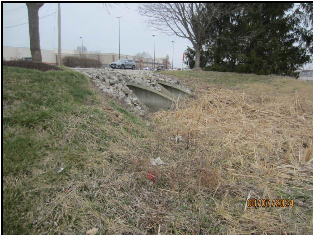
Subject Property – Looking Northwest toward RHL Drive
