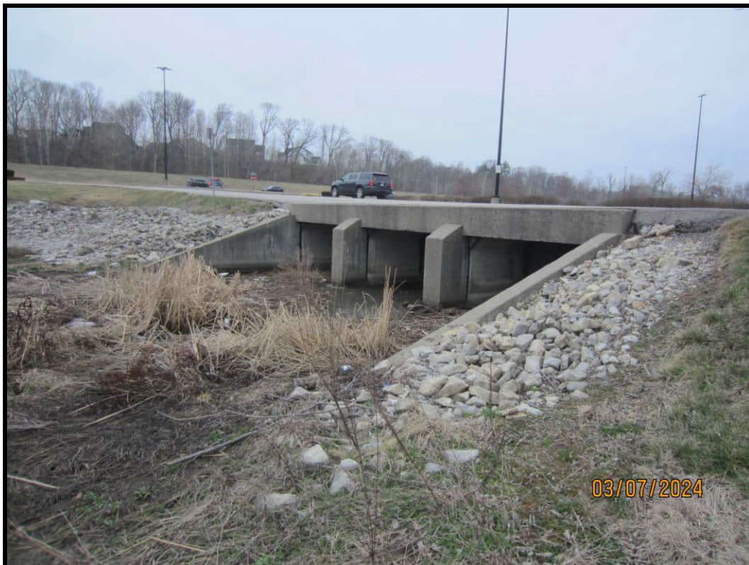
Subject Property – Looking Southwest toward RHL Drive & Edison Avenue
